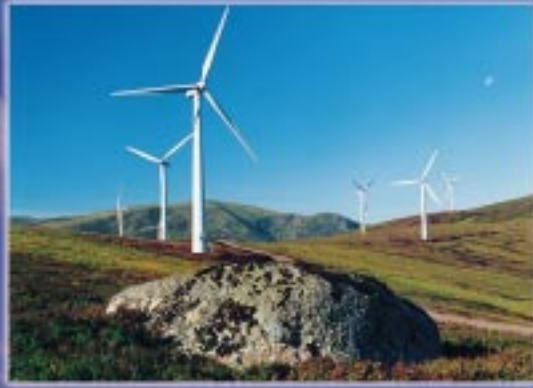
Novar Wind Farm, Scotland, by National Wind Power.
