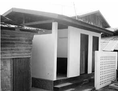
The communal toilet constructed by the community
